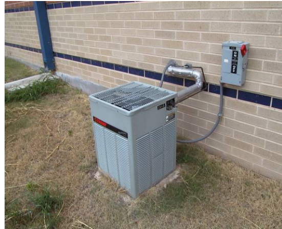
Figure 3. Air cooled chillers, and DX unit (typical) at Blattman Elementary School
