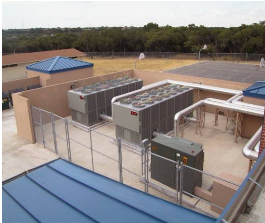
Figure 3. Air cooled chillers, and DX unit (typical) at Blattman Elementary School
